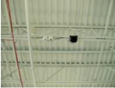
Figure 4 - SensorSwitch Daylight, Occupancy Sensors
